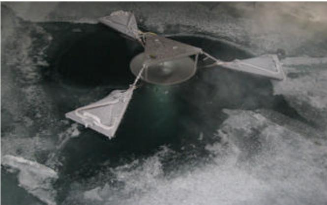
**Figure 4.** Holes can be broken through ice up to about 0.2 m thick to install a SolarBee mixer.
